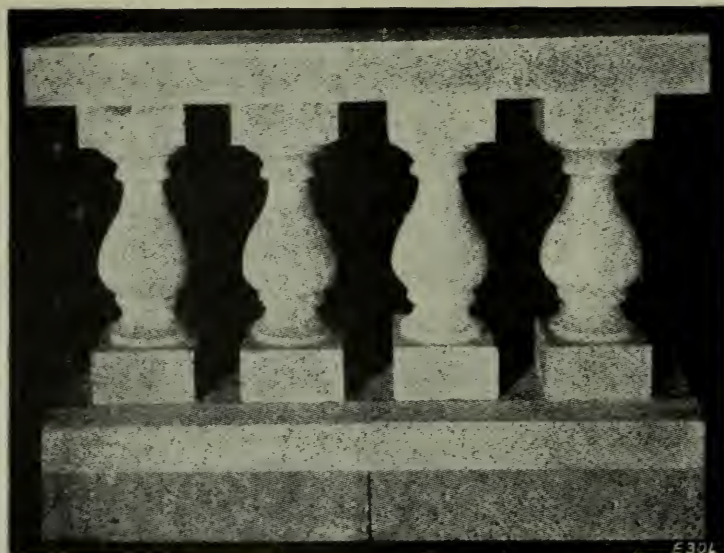
FIG. 3. CONCRETE BALUSTRADING WITH DRESSED SURFACE.
